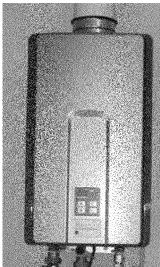
Figure 6. Japanese tankless gas water heater
